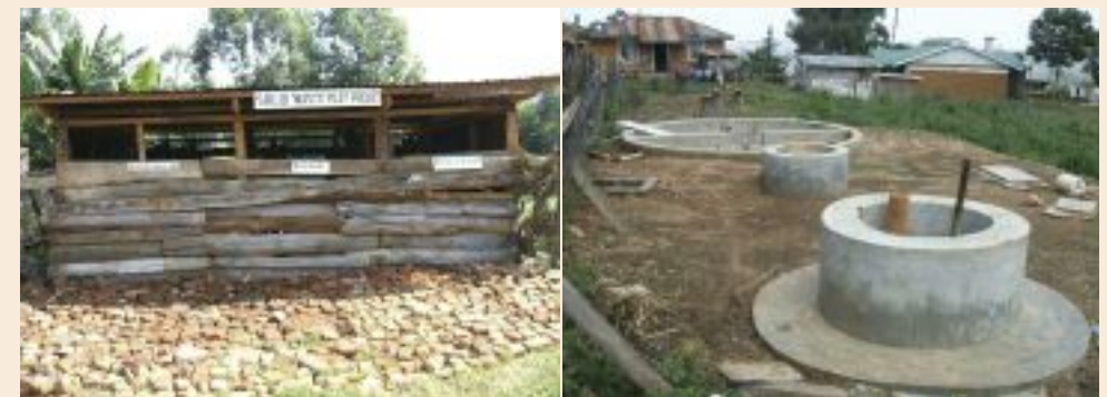
Waste is segregated at Gobei High School, while its biogas digester provides compost
